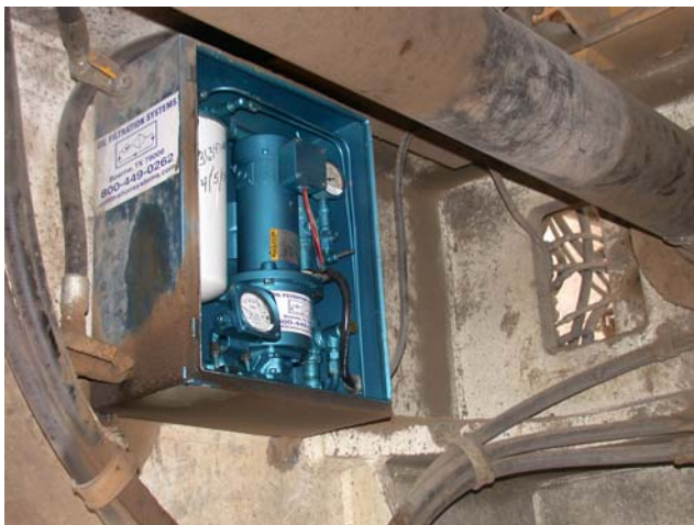
Actual On-board System with Door Removed for Inspection
