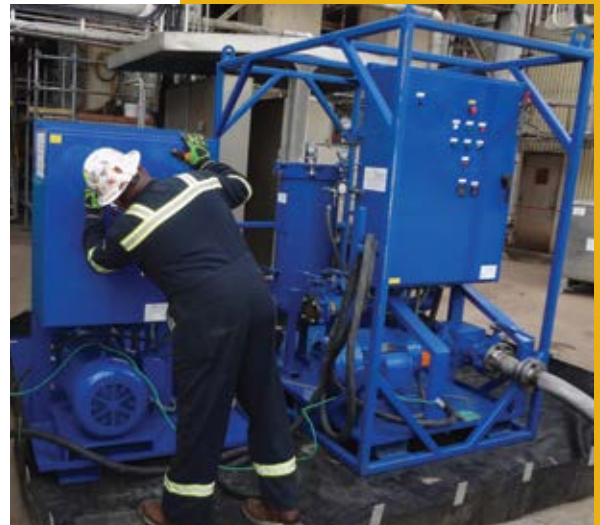
High Velocity Oil Flush of a compressor during a petrochemical plant turnaround on the Gulf Coast
