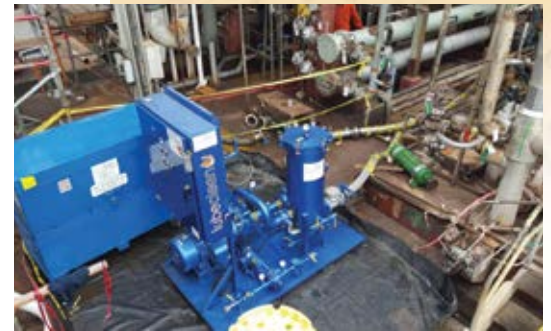
Varnish Removal Flush at a petrochemical plant in Trinidad
