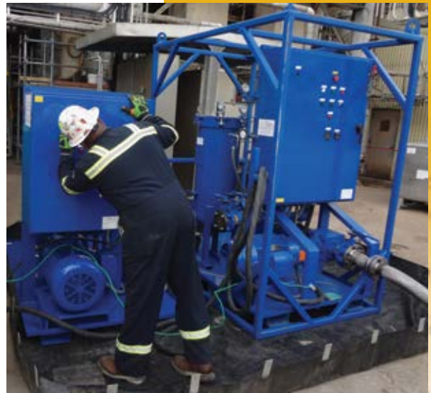
High Velocity Oil Flush of a compressor during a petrochemical plant turnaround on the Gulf Coast
