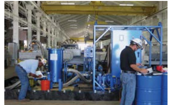
High Velocity Oil Flush of cooler bundles at a manufacturer's plant in Texas
